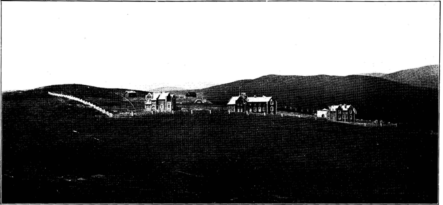
FIG. 12. ESKDALEMUIR OBSERVATORY.—GENERAL VIEW FROM THE SOUTH-WEST.
