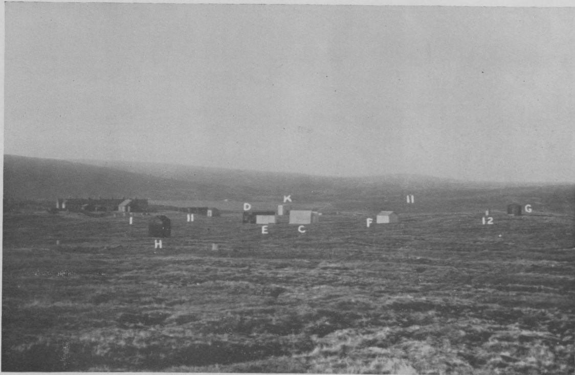
FIG. 2.—GENERAL VIEW FROM SOUTH-EAST, 1953
