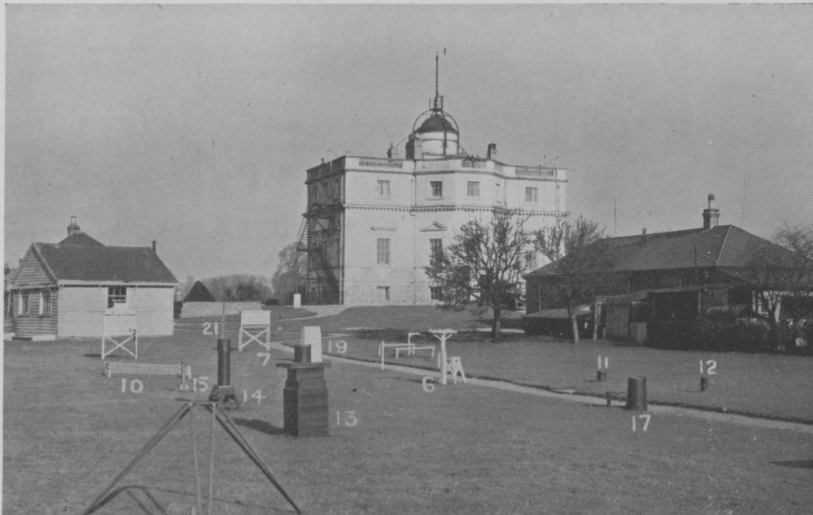
FIG. 21-GENERAL VIEW FROM SOUTH-WEST, MARCH 1953
